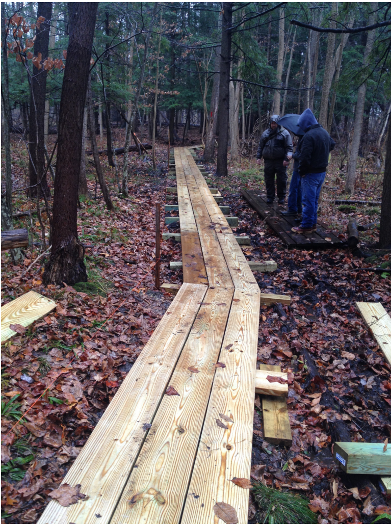
A section of boardwalk completed by the Order of the Arrow scouts on Nov. 2, 2013.
